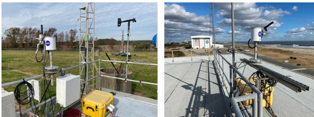
Figure 4.6.2: Michael and Steven installed Pan37 at Langley (Left) and Pan49 at Wallops.
