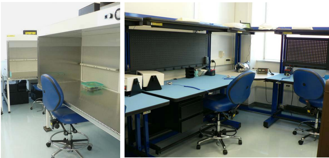
Examples of the new clean rooms (left) and laboratory facilities (right) that are now installed in Bldg. 21
